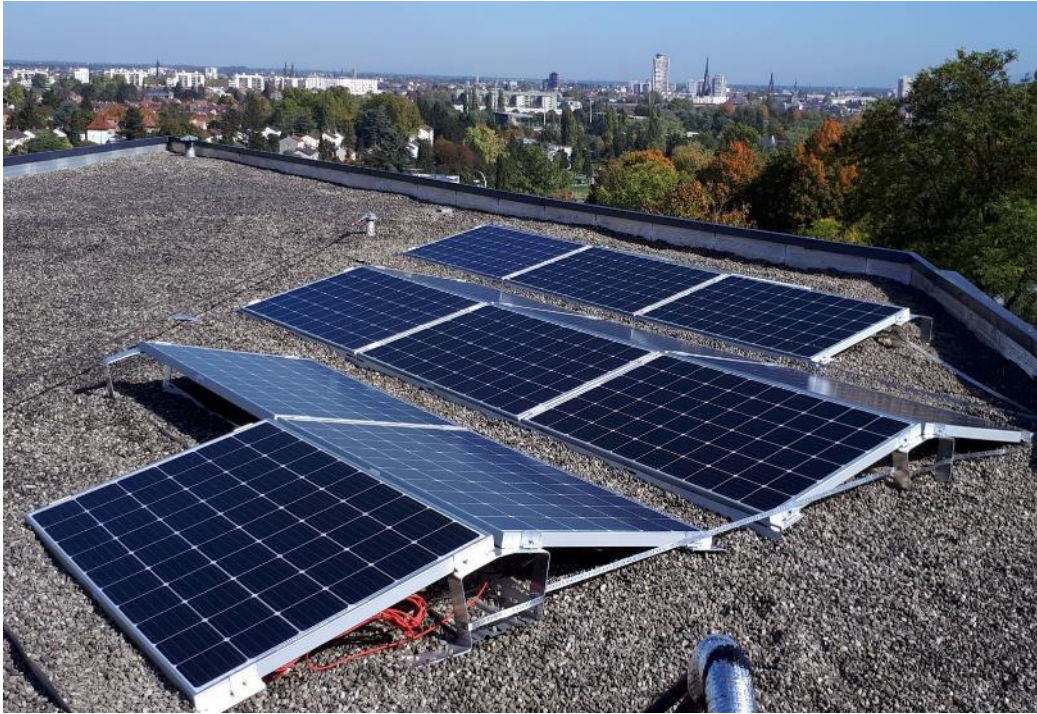
6 kwc of PV production (3 Kwc East and 3 Kwc West - ENSISA)
